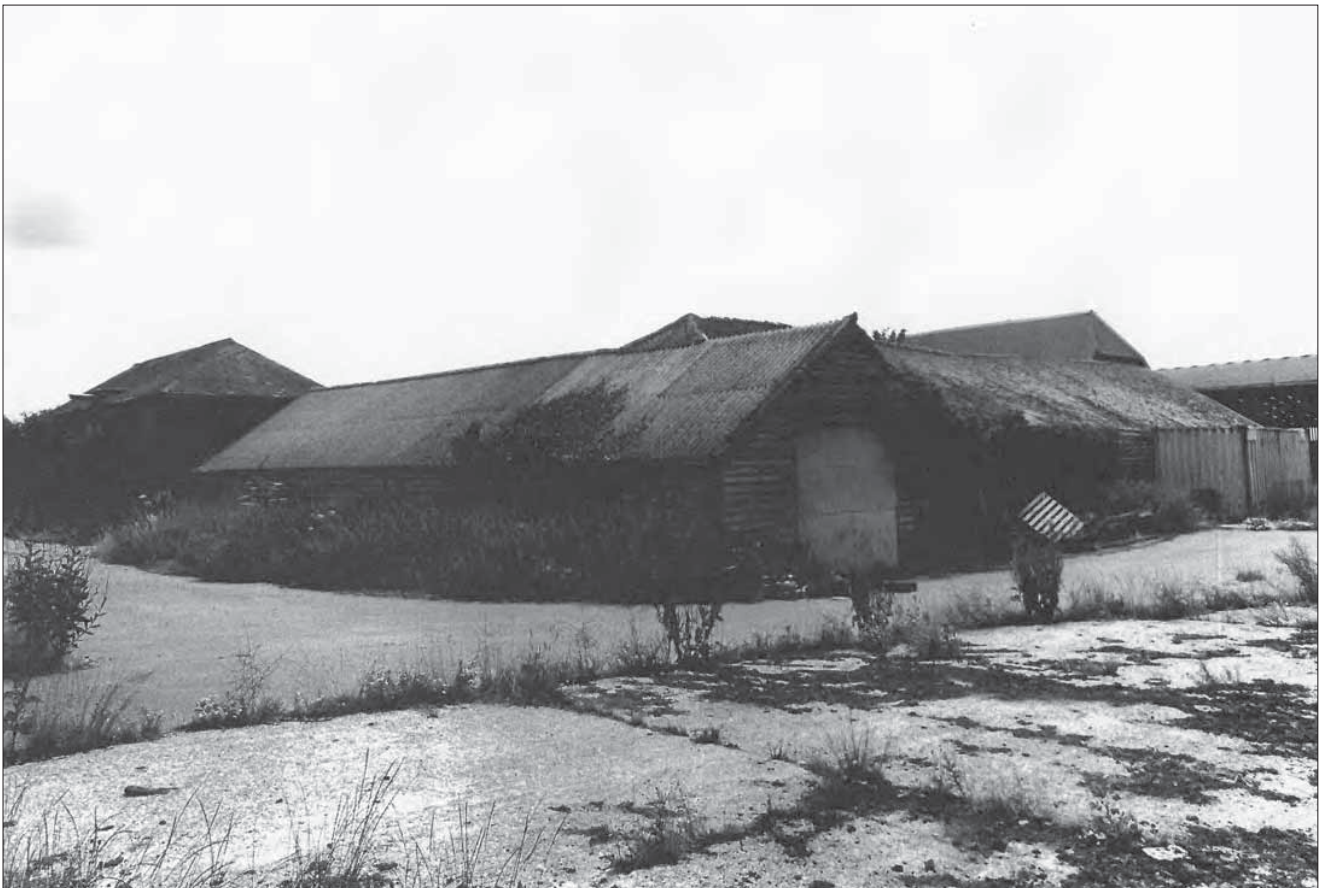
Appendix 4.11: Exterior view of the barn to the north-west of the farmyard from the north west, taken in 2000 (image slightly cropped top/bottom). © English Heritage NMR Ref.: AA030279.
