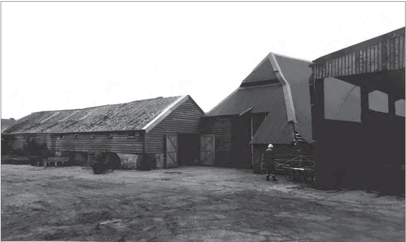
Appendix 4.3: Photo 10 of the 1988/1991 survey report, taken from the entrance to the farm and facing north-east, showing car shed (Building 10) and west end of the barn (Building 11) and corner of the dairy cowshed (Building 12). A note highlights the 'gale damaged roof' of the barn.
