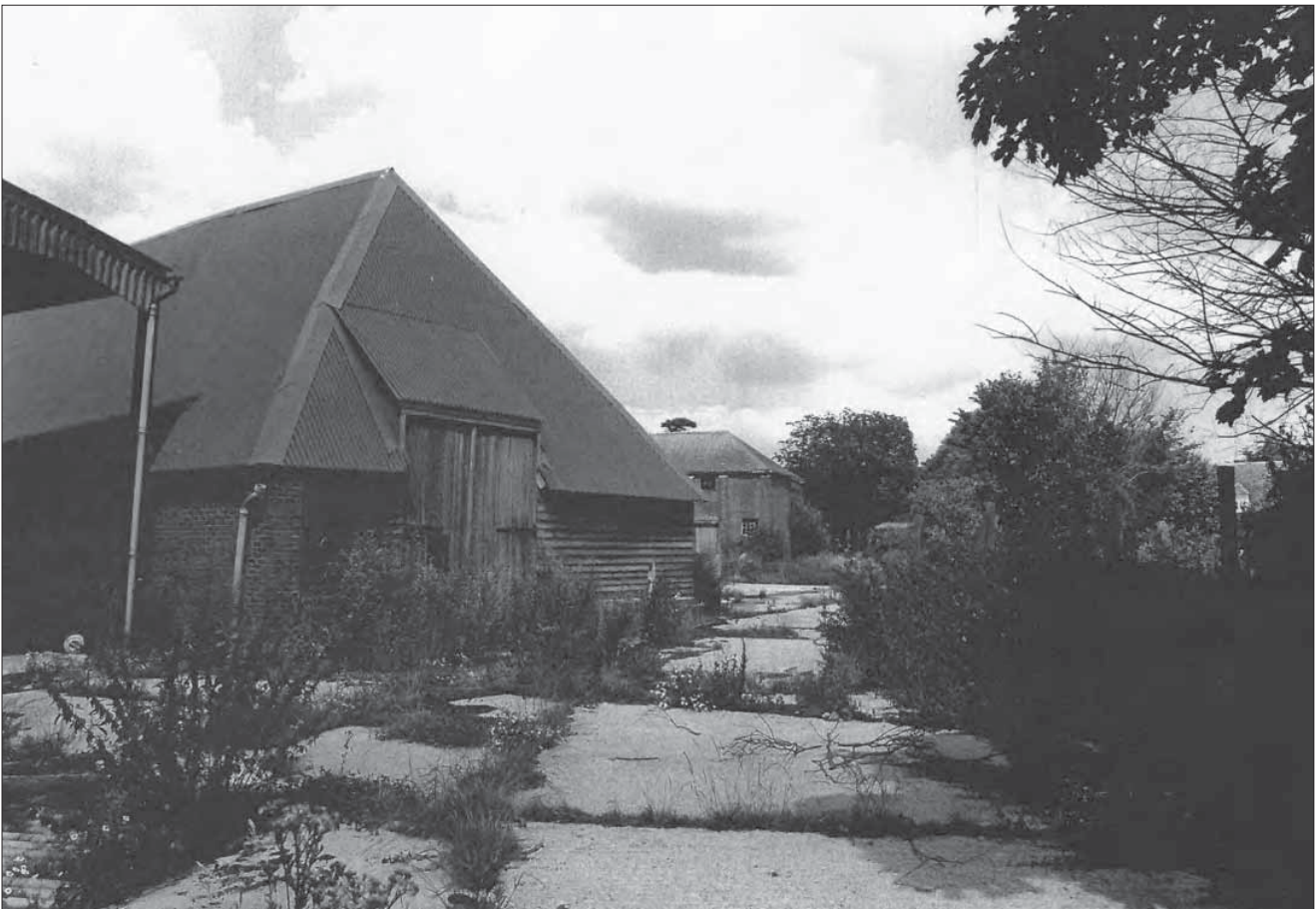
Appendix 4.5: Exterior view of the southern barn from the south-east, taken in 2000 (image slightly cropped top/bottom). © English Heritage NMR Ref.: AA030273.
