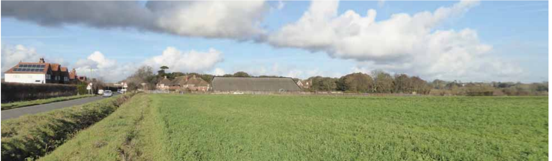
Appendix 8.6: The southern barn, seen in the middle ground from the south-west, on Posbrook Lane.
